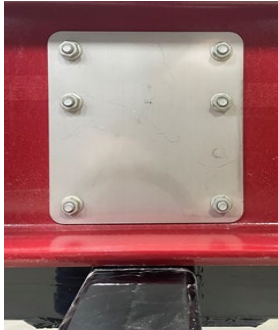
Installed (inside view)
